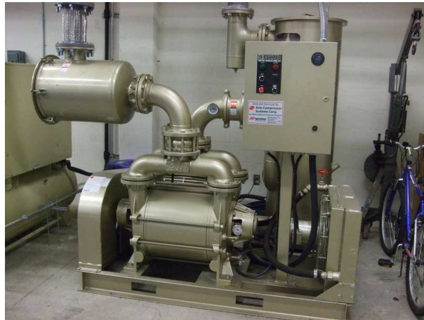
Figure 5.9: 60 Hp Vacuum Pump
