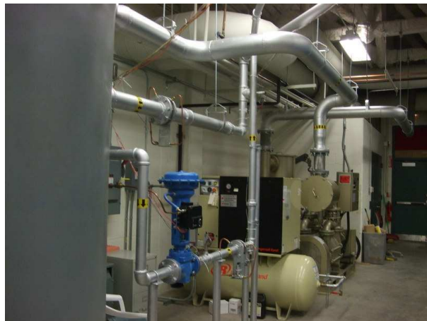
Figure 5.11: Piping for Air Delivery System
