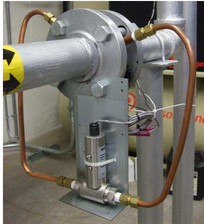
Figure 5.8: Spectre Sensors Model D150 Differential Pressure Transducer
