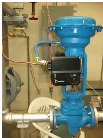
Figure 5.6: Pneumatic Computer Controlled Valve
