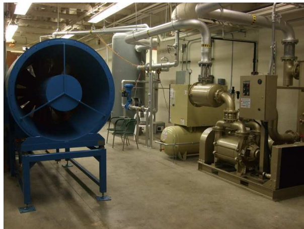
Figure 5.12: Overall View of CFJ Wind Tunnel Laboratory
